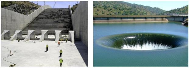
Fig. 1: stepped spillway with chute blocks, morning glory spillway
