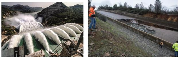
Fig. 2: spillway in operation, damaged spillway
